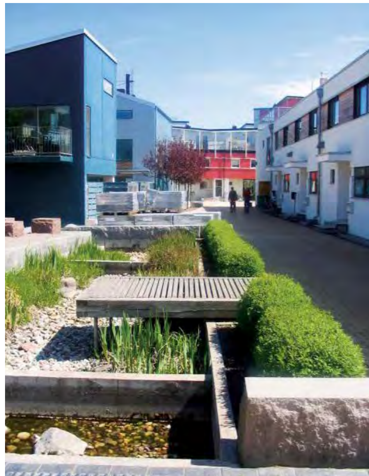
SuDS to shape street character, BO01, Malmo, Sweden.
