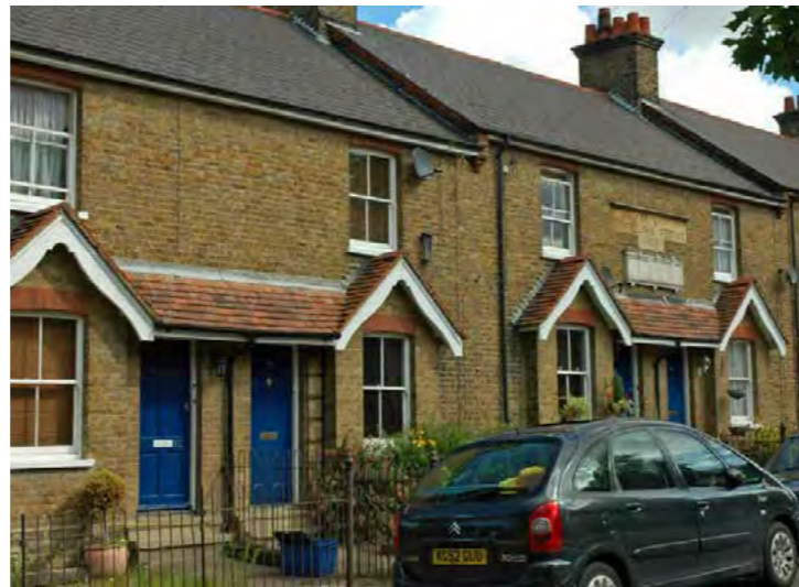
Articulated windows on Oddfellows Terrace, Old Harlow.
