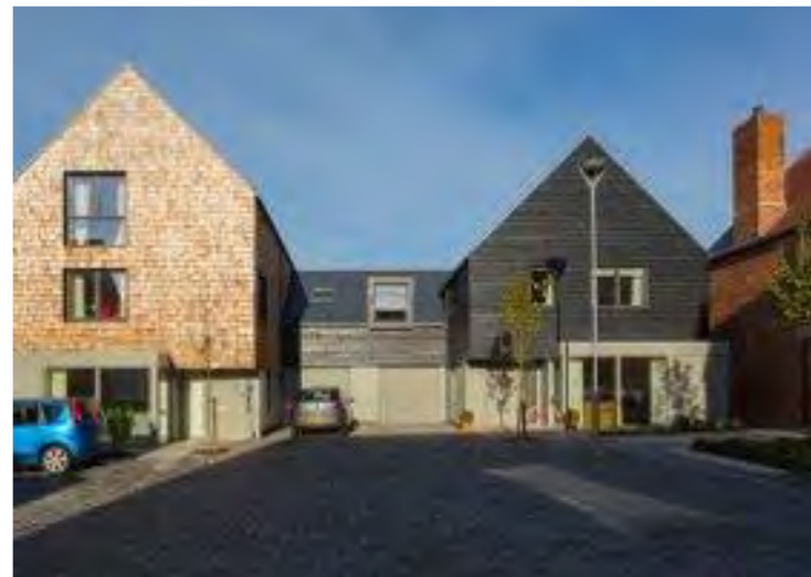
Spur street informal space example at the Avenue, Saffron Walden by Pollard Thomas Edwards Architects.
