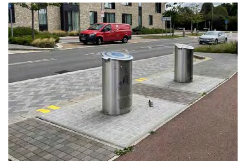
Underground refuse and recycling system, Eddington, Cambridge.
